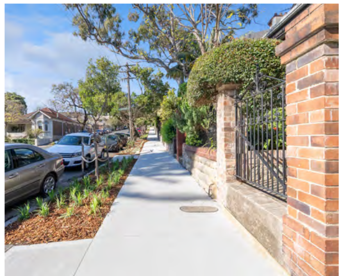
Images: Eglinton Road, Glebe Footpath Renewal Works 2021
